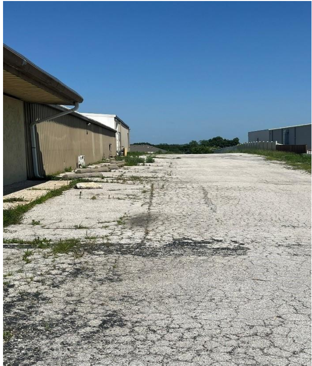
Figure 8: Deteriorated Parking Improvements
